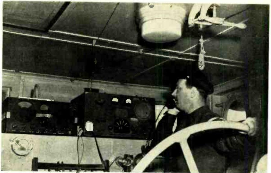
Among the best sales and service prospects are tugs and workboats. Elimination of revenue losses due to wasted time has, in many cases, paid for an installation like this in only one day's operation. Receiver at left monitors the ship-to-ship channel while the radiotelephone at right is busy on the ship-to-shore frequency. Pleasure-craft owners are also increasing use of radio, for safety and convenience.
